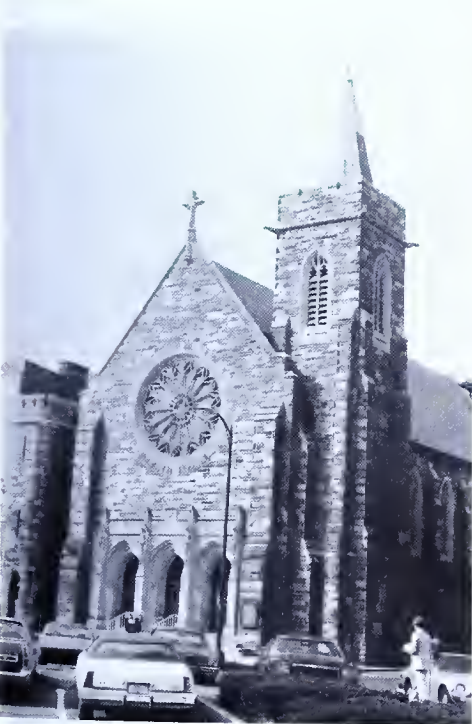
St. Lawrence Catholic Church, 108 State Street; mica schist from the Philadelphia area.
